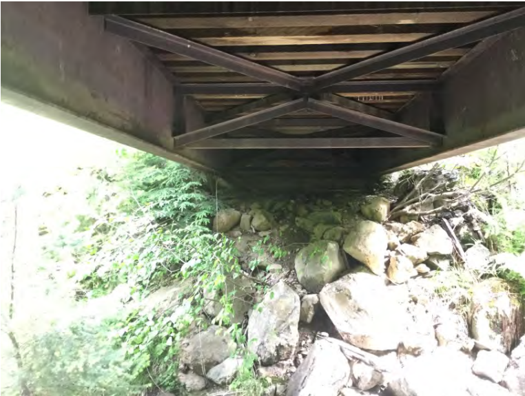
Right Bank Abutment when facing downstream
