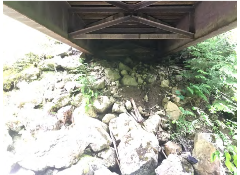
Left Bank Abutment when facing downstream
