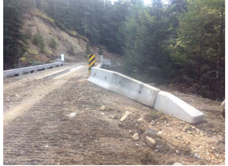
Maintenance work completed in October 2019
