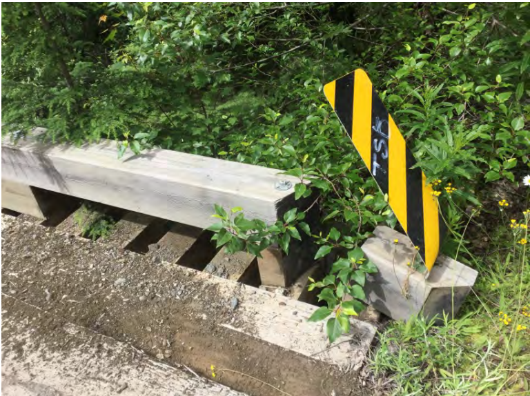
Down stream right bank rail and riser
